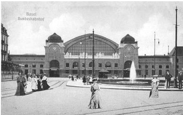
Central Train Station Basel, early 20 th century
